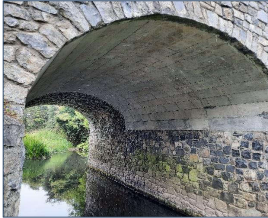
Plate 4-7 Interior bridge view
